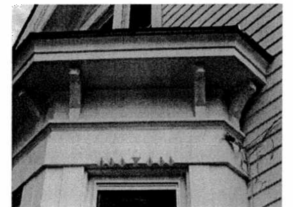
The Hazelton House is handsomely detailed with finely-crafted wooden details, including gable cross-bracing, brackets, and delicate notching on eave bargeboards and above windows and doors.
